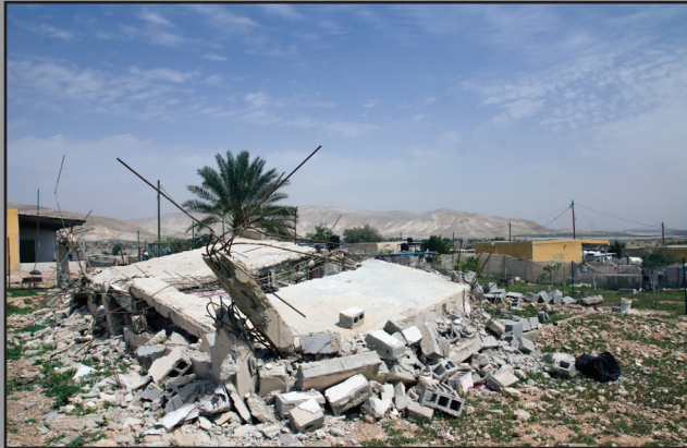
Demolished home in a Bedouin encampment, Jordan Valley, 2014 - with thanks to photographer William Parry.
