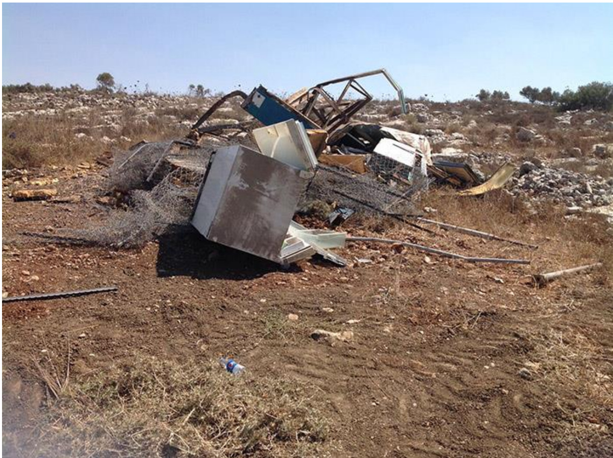
Demolition of agricultural structures in Rujeib (Nablus), 14 Sep 2022. Photo by OCHA
