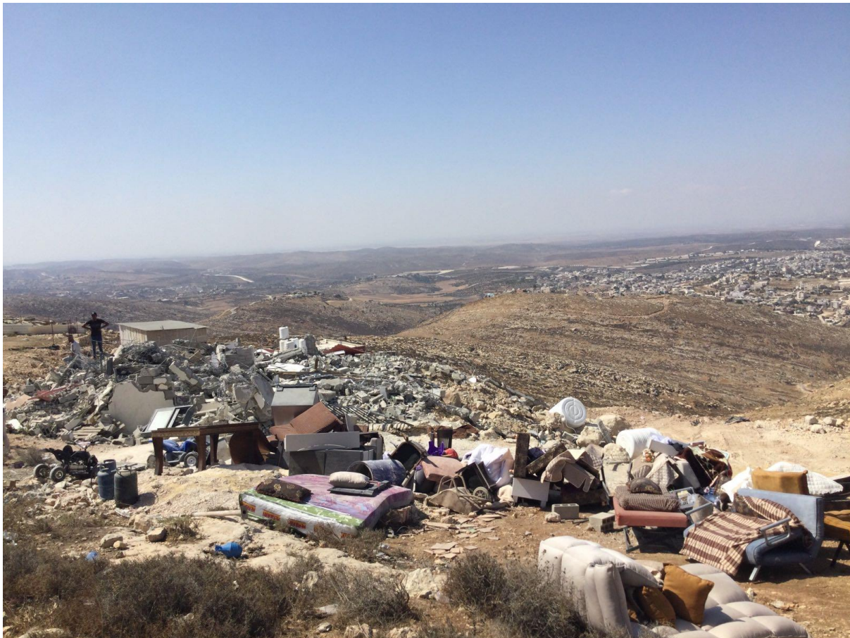
Demolition, residential house, Deir Samit, 6 October 2022
